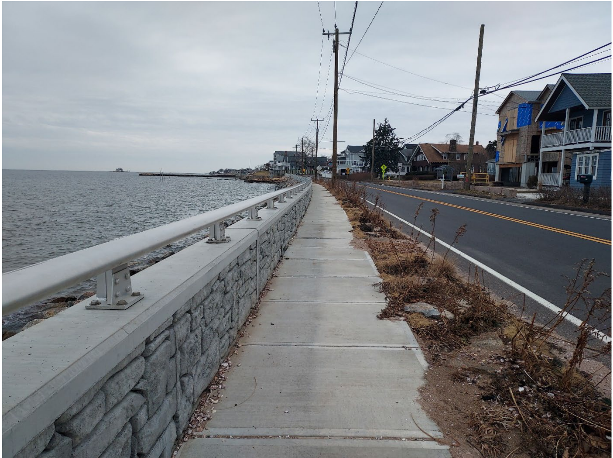
Figure 2 Limewood Ave new sidewalk and sea wall
