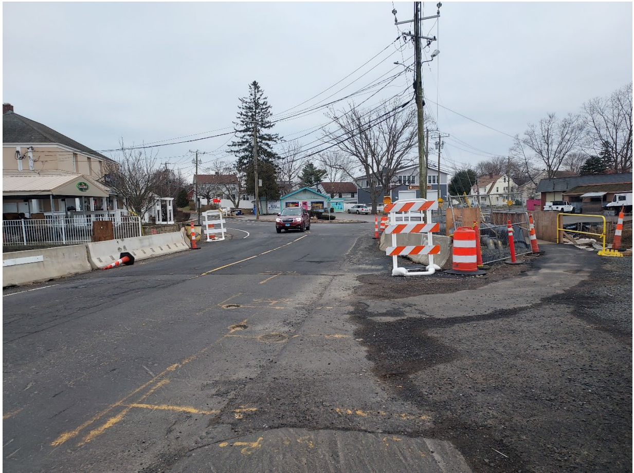
Figure 3 Sybil Creek Bridge replacement near Linden Ave (as of February 2023)
