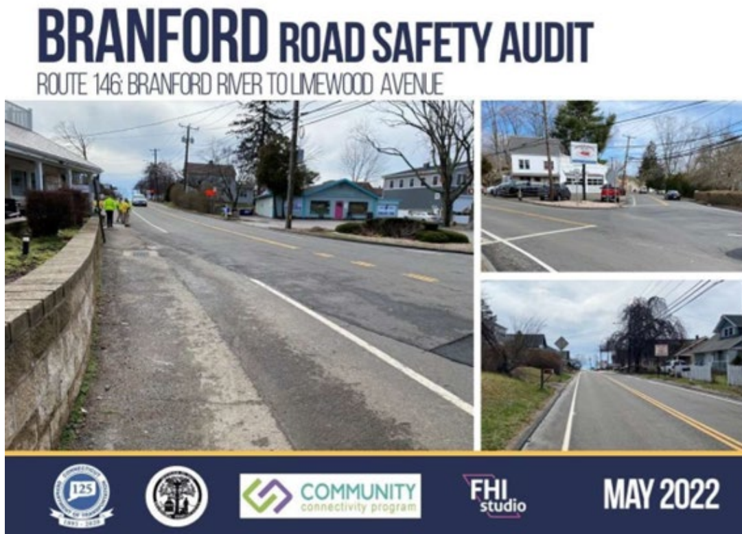
Figure 8 Cover page of Branford Road Safety Audit for Route 146
